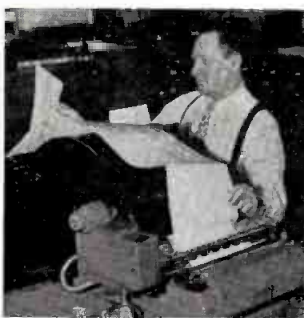
AT CBS Radio's 55 E. 52nd St. offices, William G. Stolzenberg, manager, network tabulating department, checks results as printed by IBM's tabulator (model 405). The tabulator is only one of a battery.
